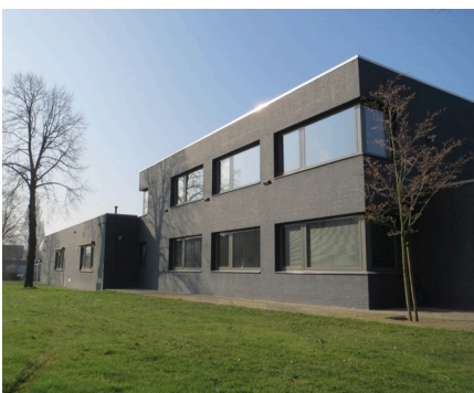
ebm-papst Heating Systems in s'Hertogenbosch (Holland)
