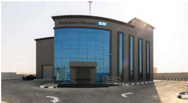
Endress+Hauser has opened a calibration and training center in Jubail, Saudi Arabia.
