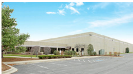
To meet the challenges of the market and to increase its own production capacity, FMI has decided to use additional facilities for clean-room production. The company moved into new 6,500 m 2 headquarters close to the former production site in Chicago and constructed an ISO Class 7 clean room with a surface area of approx. 1,900 m 2 there. (Source: Flexan)
