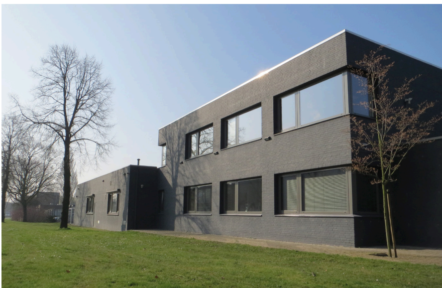
ebm-papst Heating Systems in s’Hertogenbosch (Holland)
