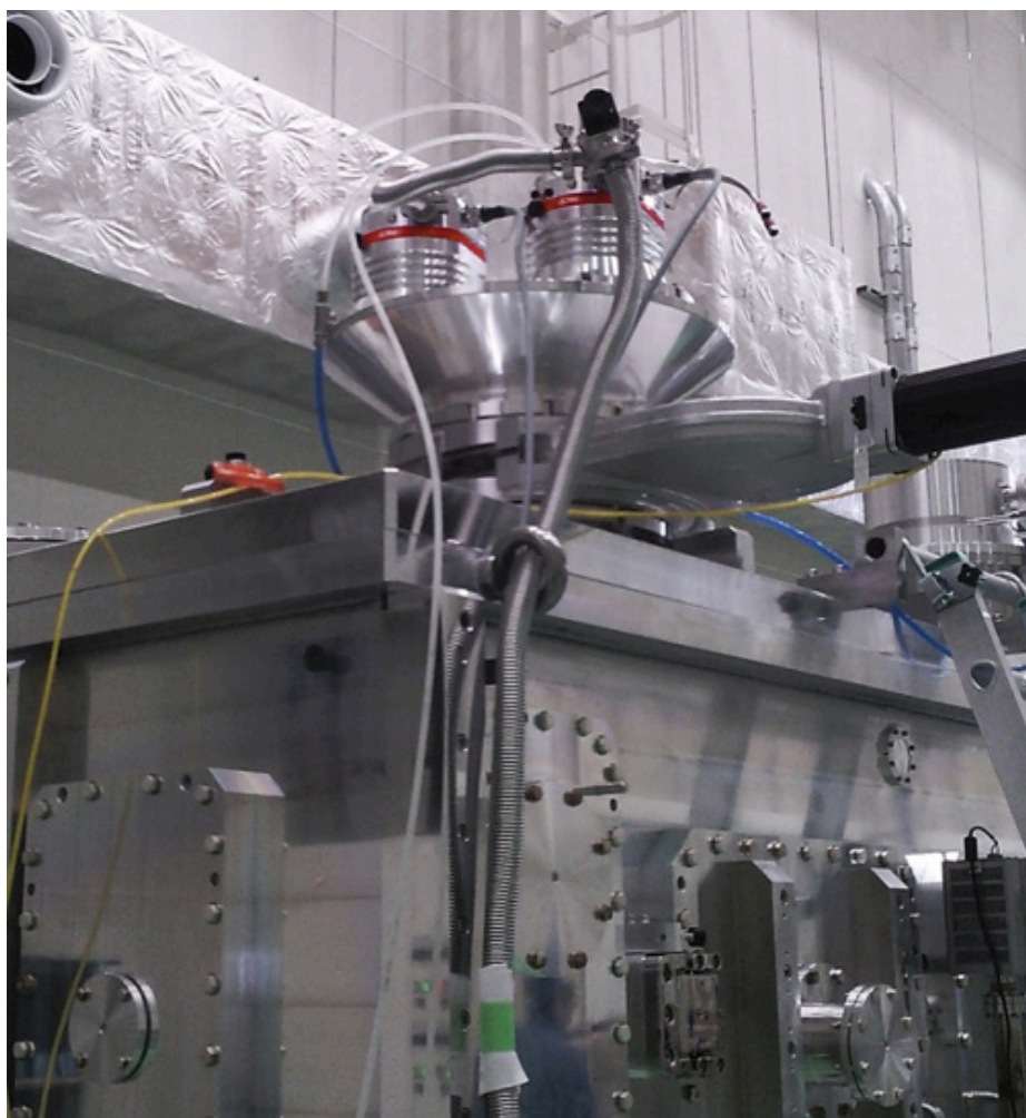
HiPace turbopumps installed at XFEL
