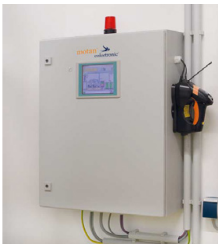
The scanner is used to record bin changes and for entering the material and batch codes of the new octabins. (Photo: motan-colortronic)
